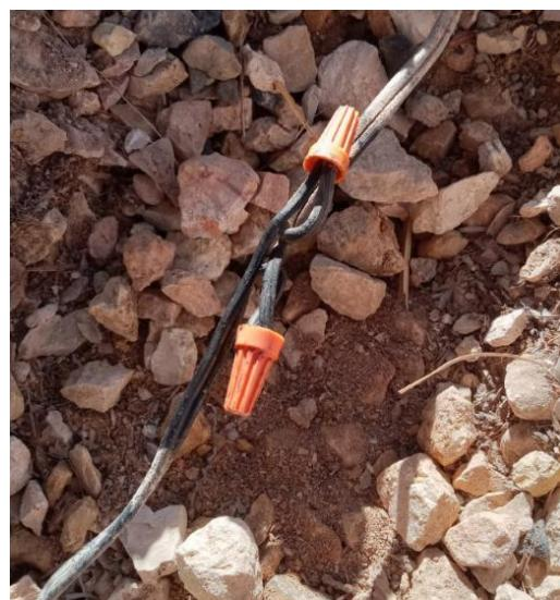
Or, you may see even more strange connections – like this example where two runs of wire were joined by a connector meant to attach lights to the wire run. Needless to say, these should ideally all be converted to soldered joints to improve reliability and increase light brightness.
