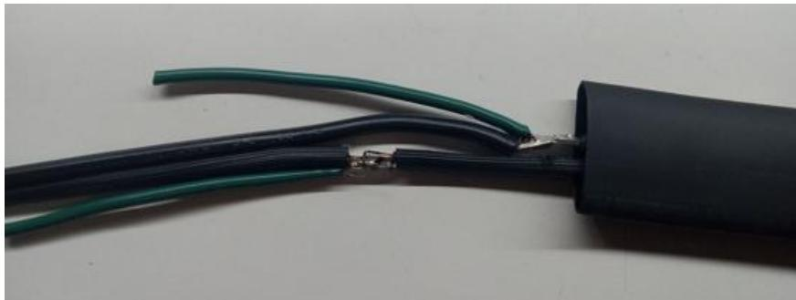
Finally slide the heat shrink over the connections and permanently apply it using a heat gun.
