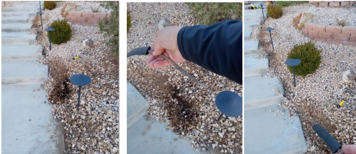
You can then use a wire stripper tool to pull back the wire insulation (without cutting the wire) on the two locations (below left.) Then flux, solder and heat shrink seal as before. Repeat for each lamp.
